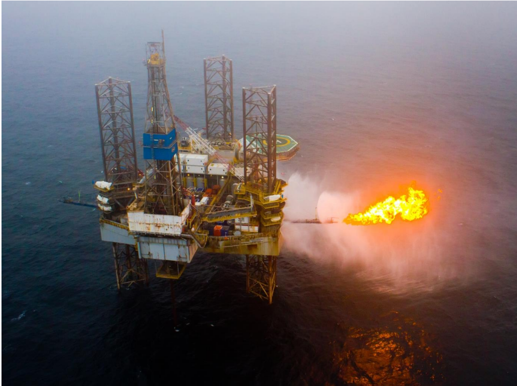
Figure 1.3 — Image of flaring during one of the isolated well tests for the Pegasus West 43/13b-7 well Q3 2014.
